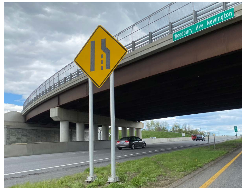
Spaulding Turnpike, Newington, NH.
